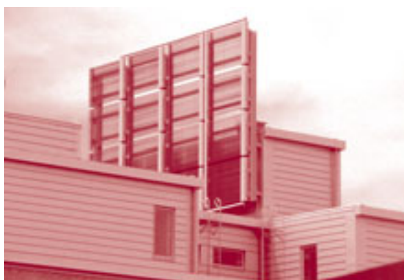
Solaranlage / Solar water heating © Jan Erik Andersson
